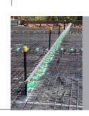
Diamond™ Dowels comply with the requirements of TR34 (4th Edition) providing load capacity at joint width gaps up to 20mm.
